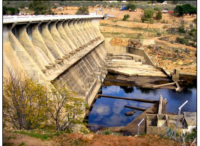
Figure 1.4 Apron below Dam wall
