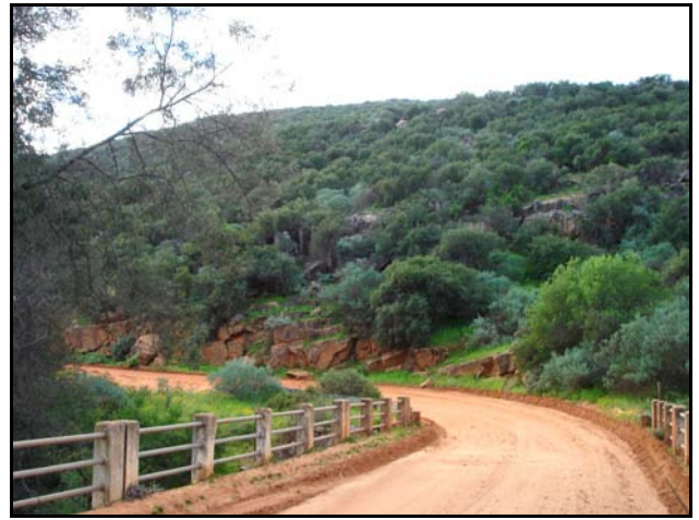
Figure 10.6 The bridge over the Rondegat River, road DR 2183
