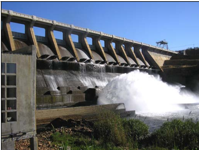
Figure 1.5 Clanwilliam Dam outlet
