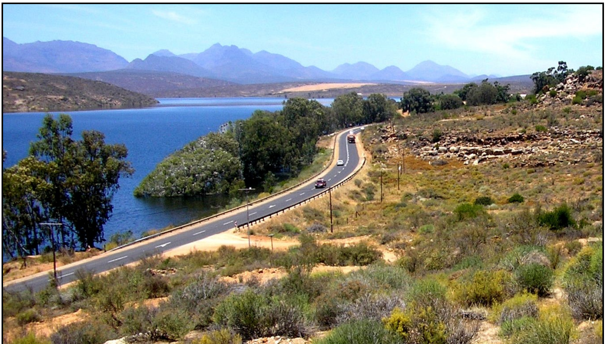
Figure 10.1 The N7 to the west of the Dam
