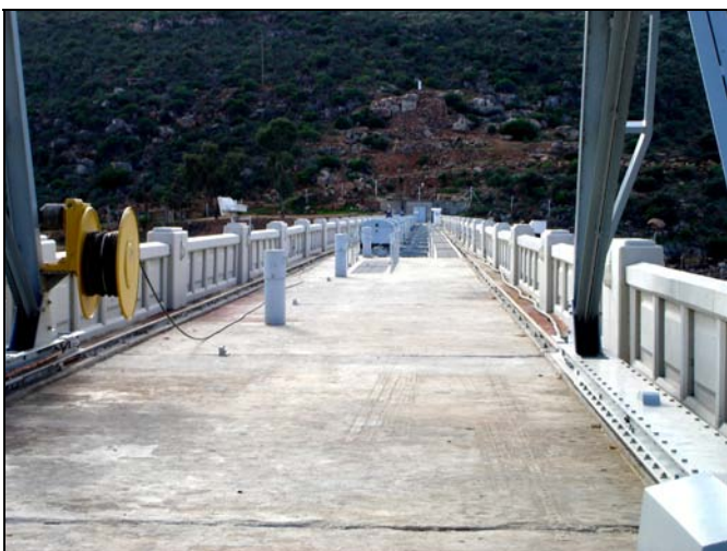
Figure 1.7 Dam wall crest
