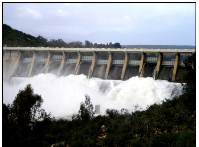
Figure 1.8 Three sluices open
