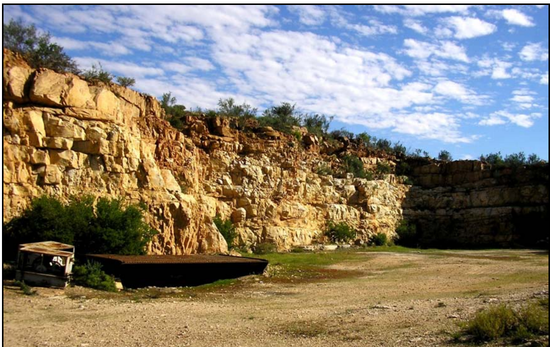
Figure 9.1 Existing quarry to the west of the Dam
