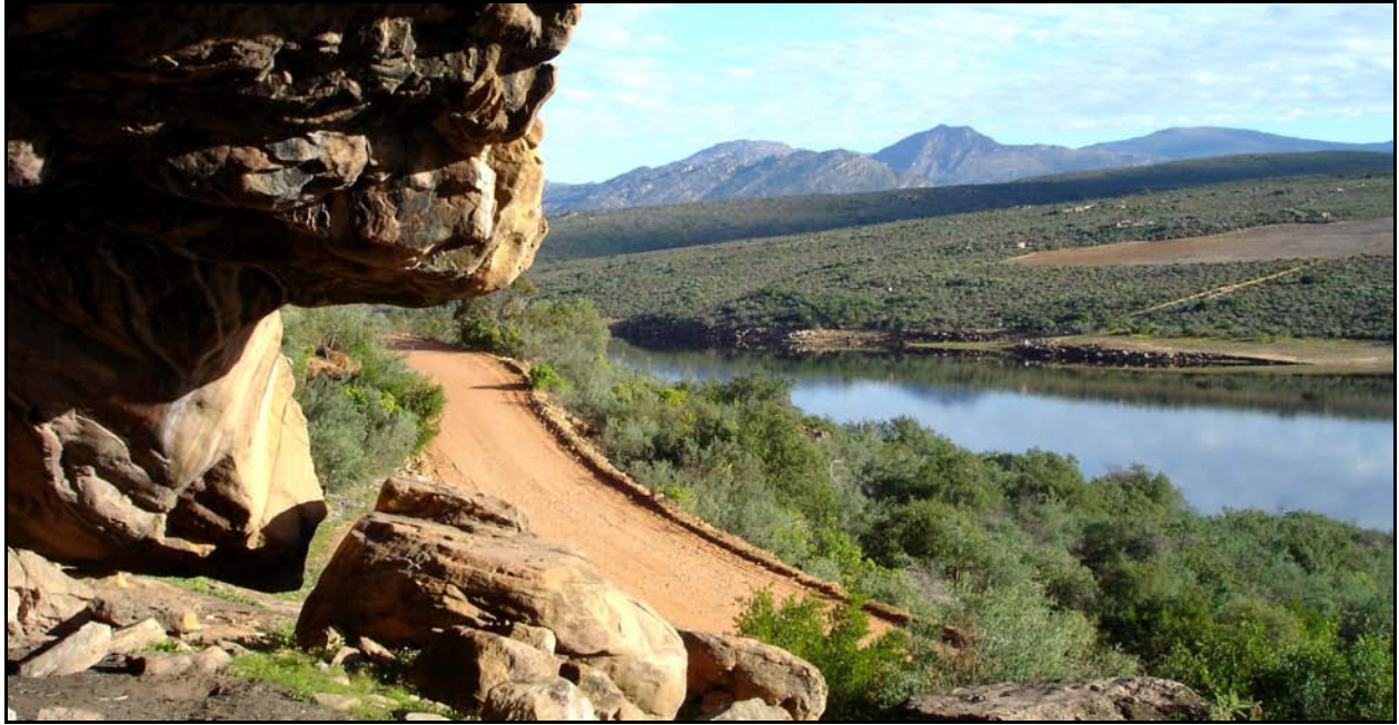
Figure 10.2 Divisional Road 2183 to the east of the Dam
