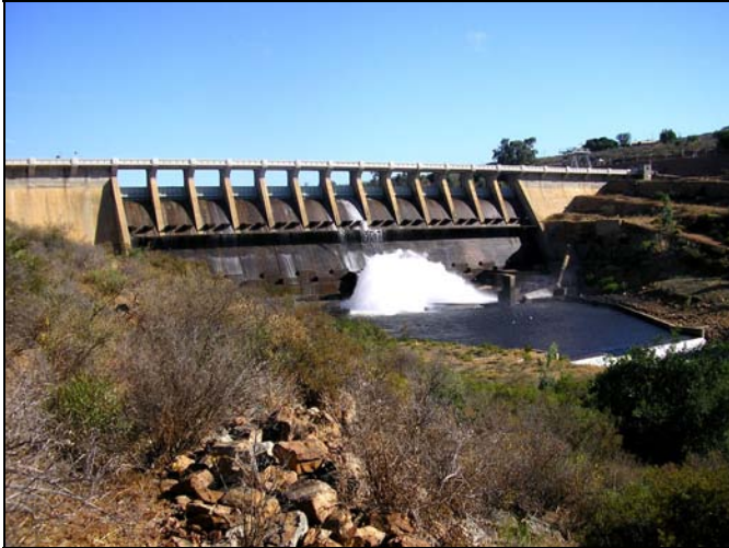
Figure 1.3 Clanwilliam Dam downstream from right bank
